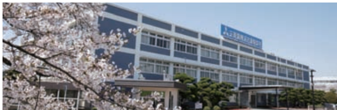
Mitsubishi Electric Nagoya Works
